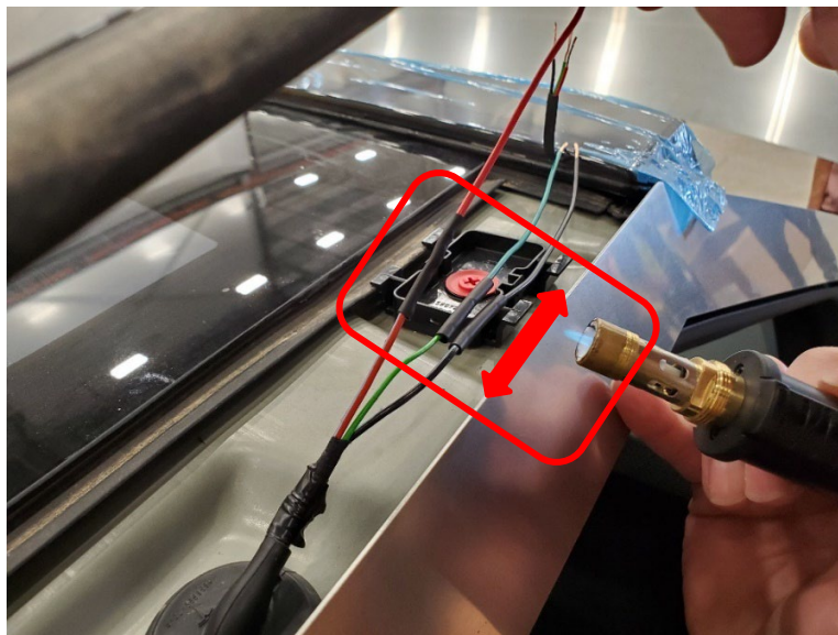
Figure 18 – Correct heat application TESLA
