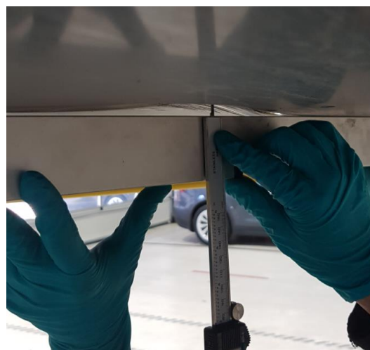
Figure 12 – Dent exceeding the maximum threshold
