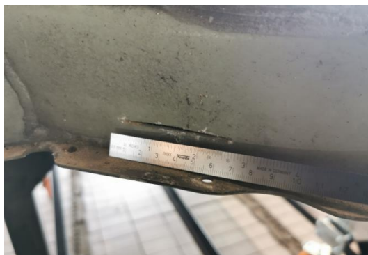
Figure 5 – Large enclosure crack breaking the enclosure sealing
